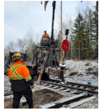
Maintenance of Way removing the hand operated switch
