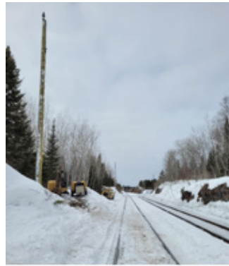
New pole line being built
