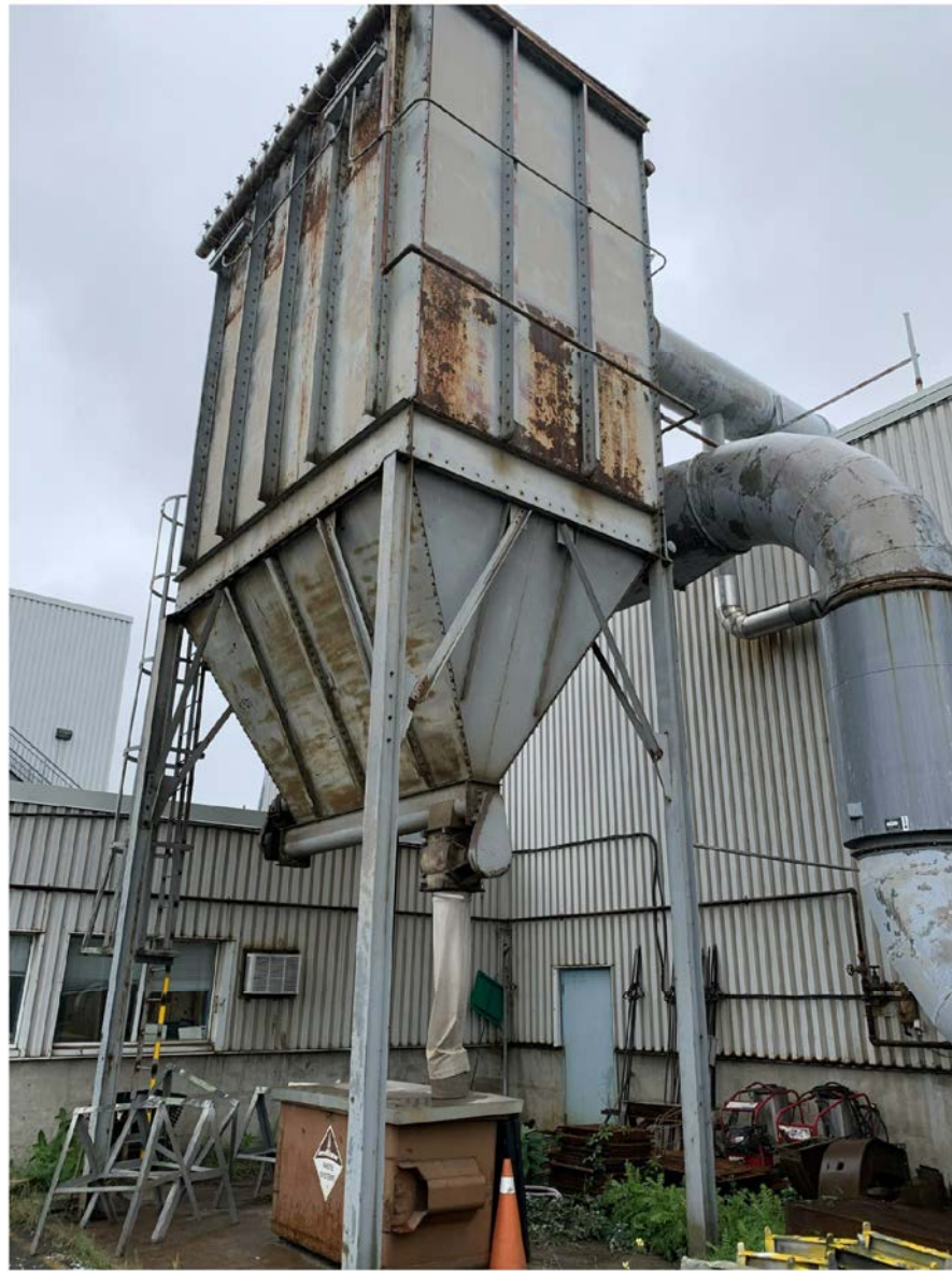
PHOTO A - EXISTING DUST COLLECTOR.
