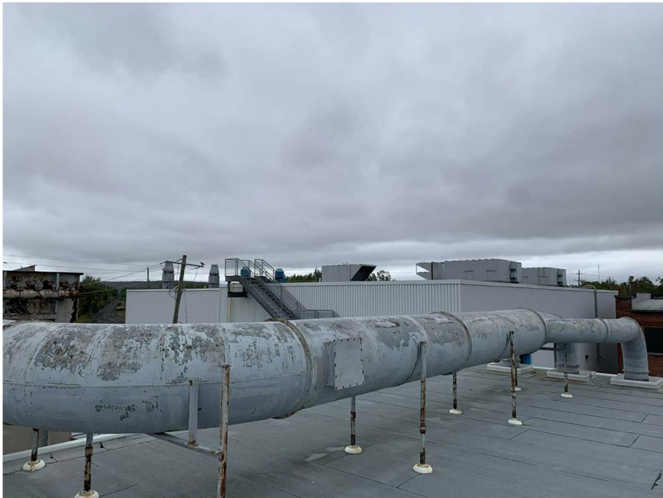
PHOTO G - EXISTING DUST COLLECTOR DUCTWORK.
