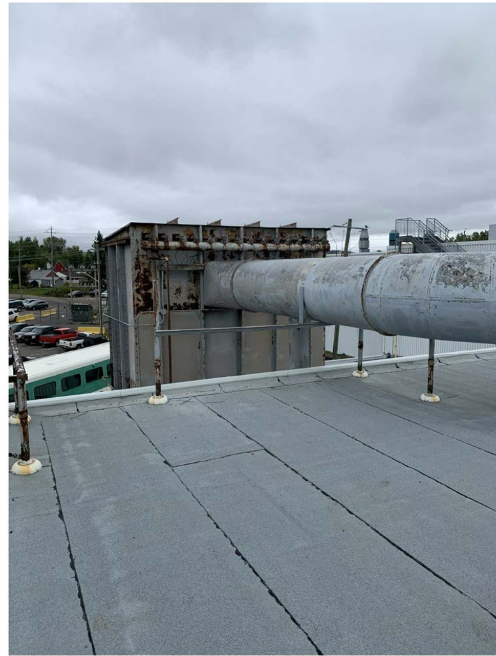
PHOTO E - EXISTING DUST COLLECTOR (HIGH LEVEL).
