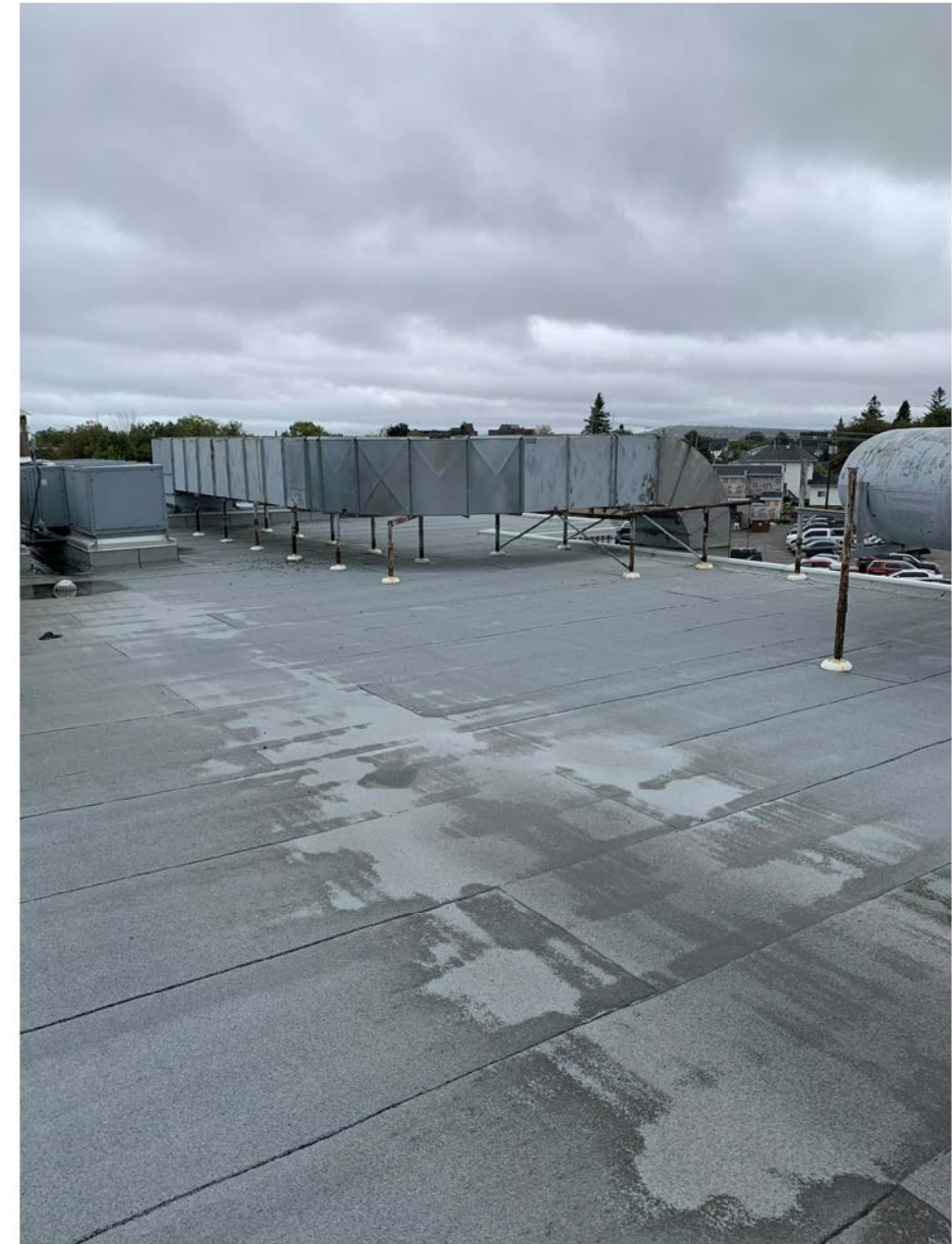
PHOTO F - EXISTING DUST COLLECTOR DUCTWORK AND GAS FIRED ROOFTOP AIR HANDLER / HEATER.
