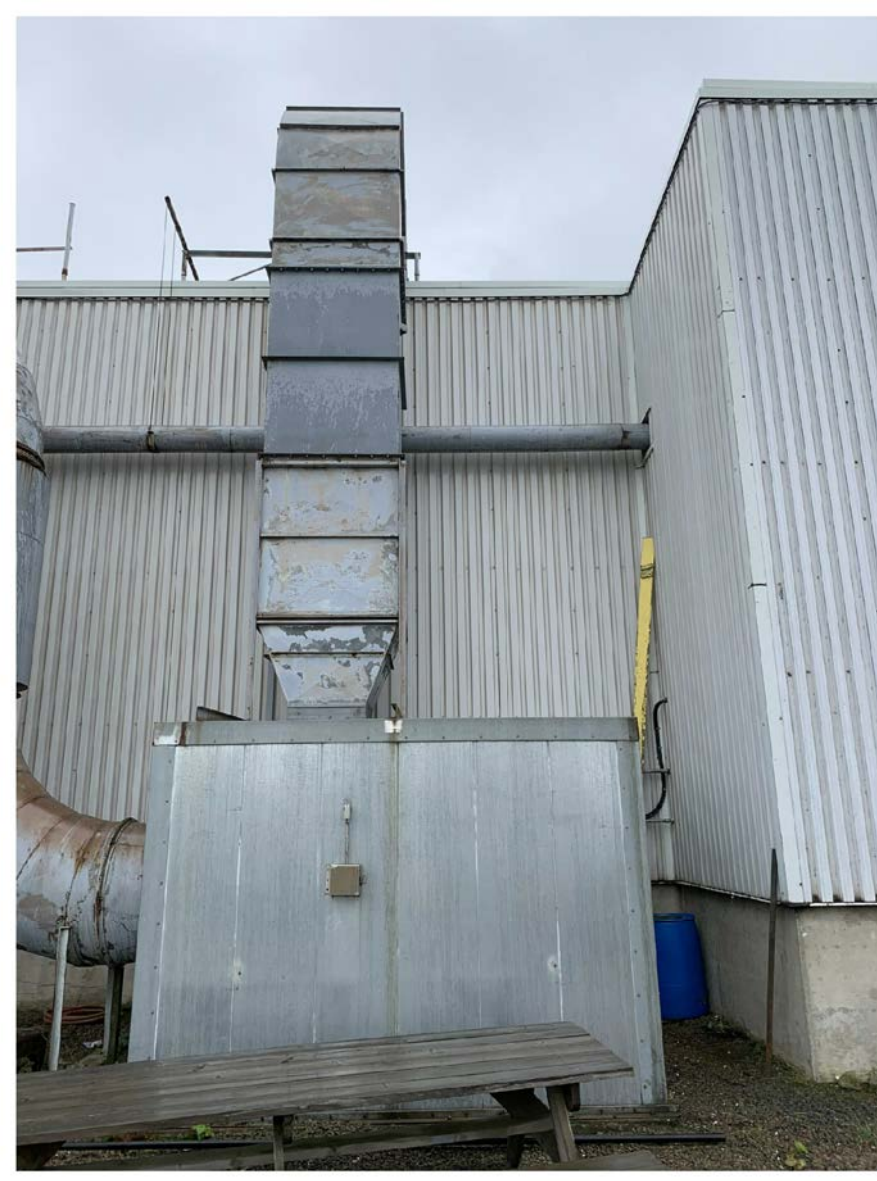
PHOTO B - EXISTING DUST COLLECTOR FAN CABINET.
