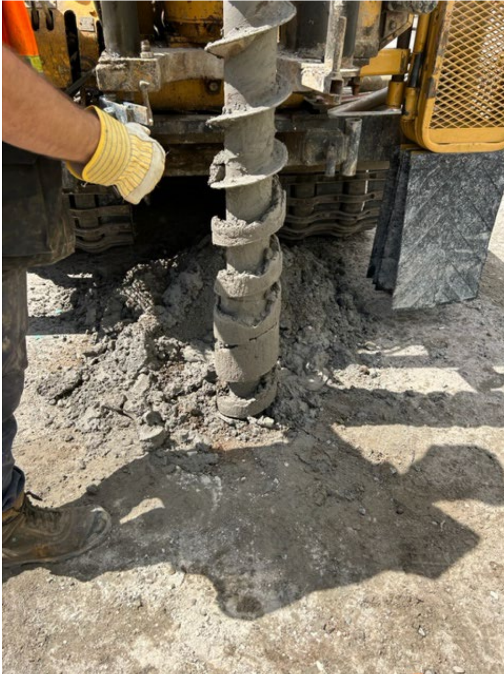
Wet Sandy silt soil
