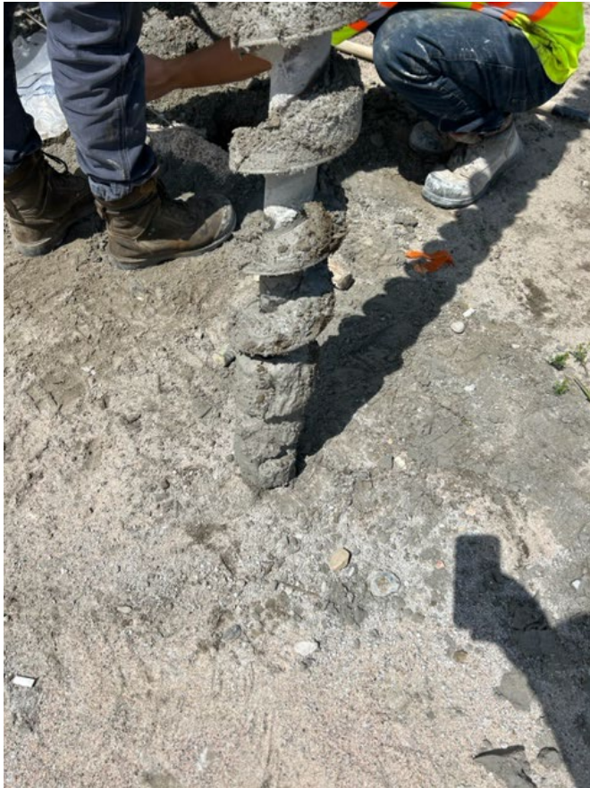
Photo #3- Saturated sandy silt at 5.5 m depth -BH-03
