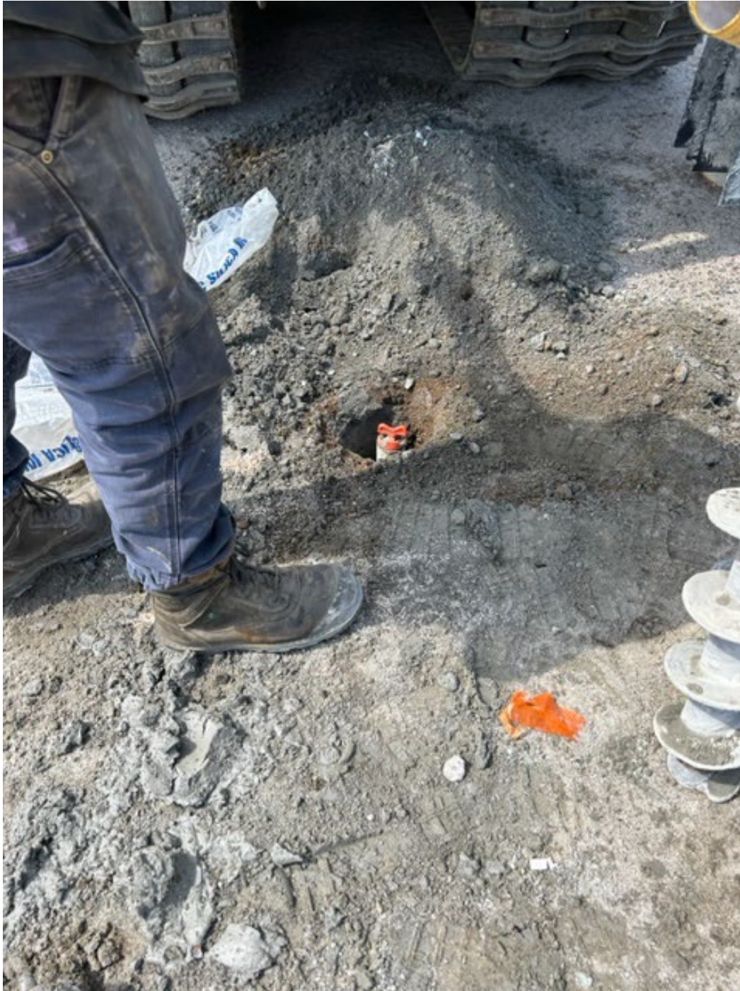
Well Monitoring Borehole #3.
