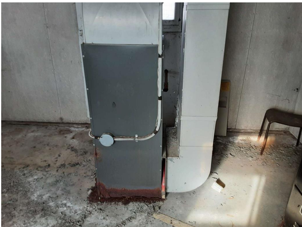
Mechanical Equipment, Furnace, Not Insulated, Main Office (Location #: 1)
