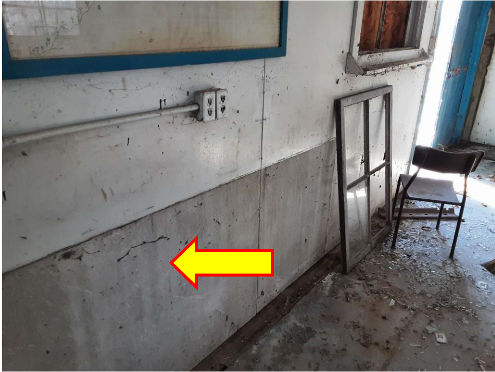
S0001A (Confirmed Asbestos), Wall, Cement Product, Main Office (Location #: 1)
