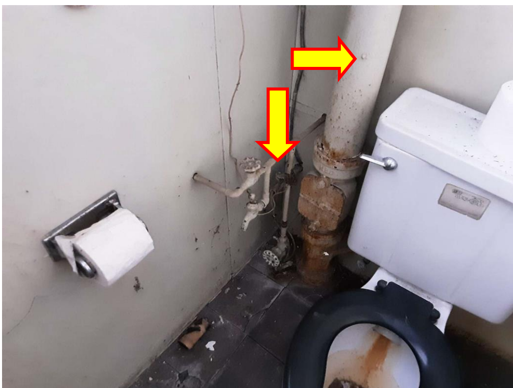
Piping, Not Insulated, Washroom (Location #: 5)
