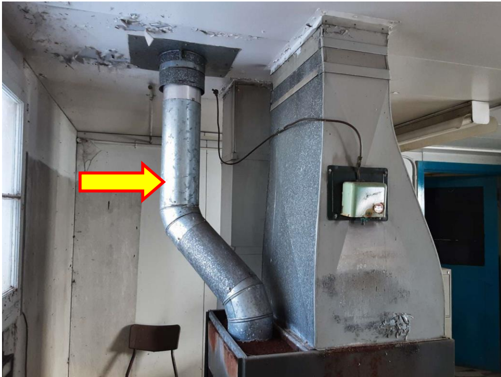
Duct, Not Insulated, Main Office (Location #: 1)
