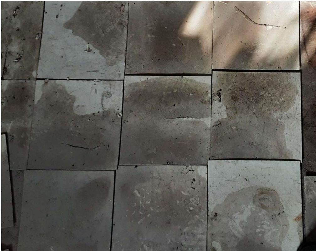
S0005C (Confirmed Asbestos), 12" x 12" white Fleck, Floor, Vinyl Floor Tile, Office (Location #: 3)
