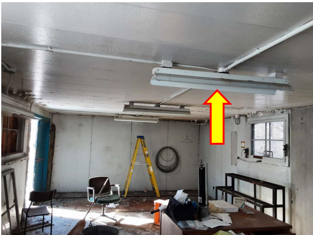
PCB, V9500(Presumed), LIGHT BALLASTS, Main Office (Location #: 1)
