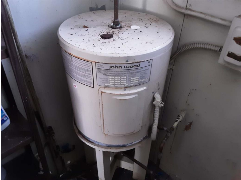
Mechanical Equipment, Heating Water Tank, Fiberglass (metal covering), Washroom (Location #: 5)
