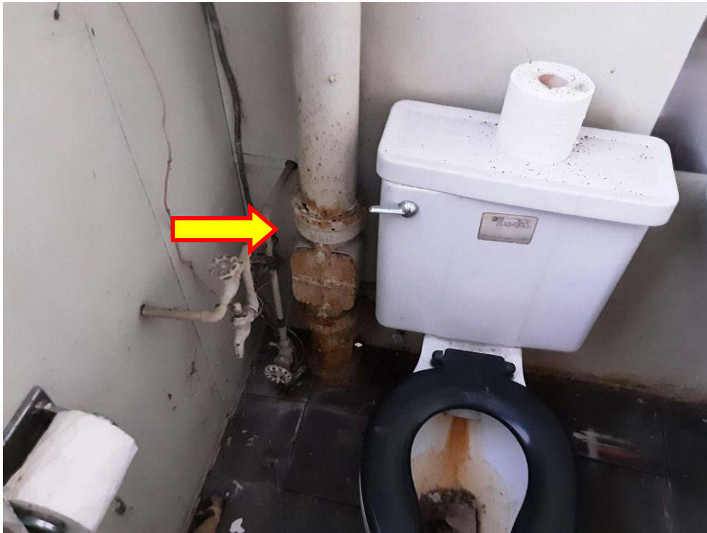
Pb Products, V9000(Yes), BELL AND SPIGOT FITTINGS, Washroom (Location #: 5)
