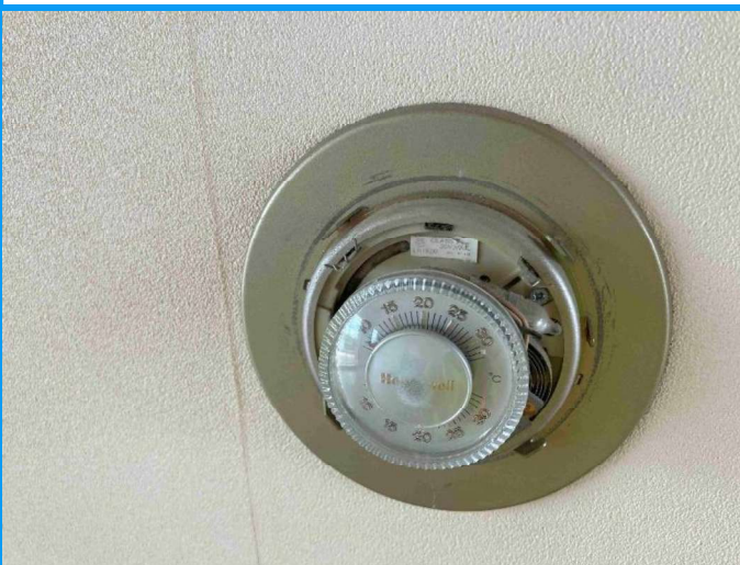
Photo 8: Typical view of a mercury containing thermostat that was observed in various areas of the subject building.
