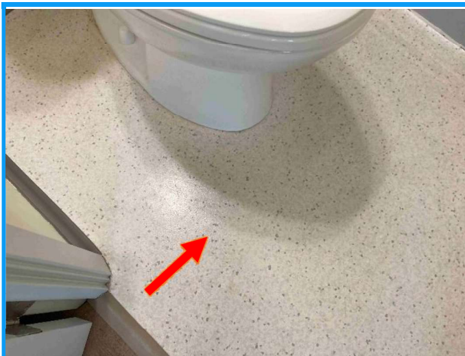
Photo 5: Typical view of the non-asbestos-containing grey with coloured mosaic pattern vinyl sheet flooring (see arrow) observed in the washrooms of the motel section of the subject building.
