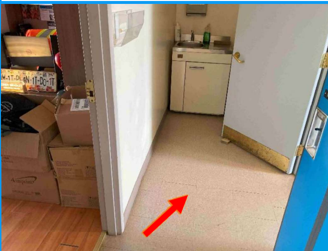
Photo 4: View of a portion of the non-asbestos containing 12"x12" Armstrong brand grey with lighter grey and white specks vinyl floor tiles (see arrow) in the ground floor corridor behind the waiting area.
