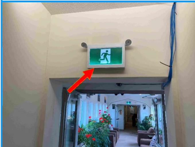
Photo 11: Typical view of an emergency light fixture (see arrow) presumed to contain a lead acid battery.
