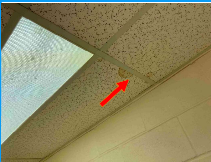
Photo 9: View of two (2) water-stained 2'x4' Dense Pinhole w/Circular Random Fissures (see arrow) in the Female Staff Locker B.13.
