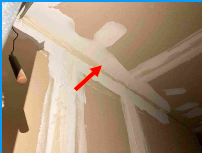
Photo 3: View of a portion of the ceiling space above the false ceiling in the 2 nd -floor corridor of the motel, featuring non-asbestos drywall walls and ceiling (see arrow).
