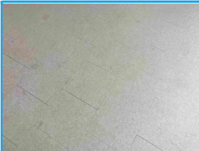
Photo 5: Close-up view of the non-asbestos-containing 12"x12" Armstrong brand grey with lighter grey and white specks vinyl floor tiles that were observed throughout the subject building.
