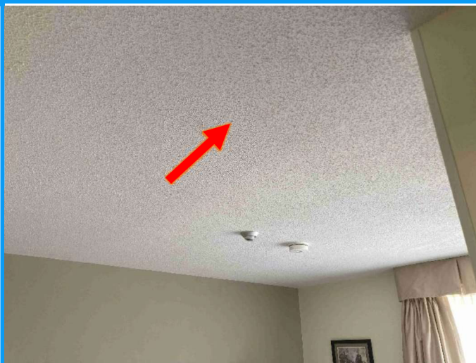
Photo 1: Typical view of the non-asbestos textured ceiling finish (see arrow) observed throughout the motel section of the subject building.
