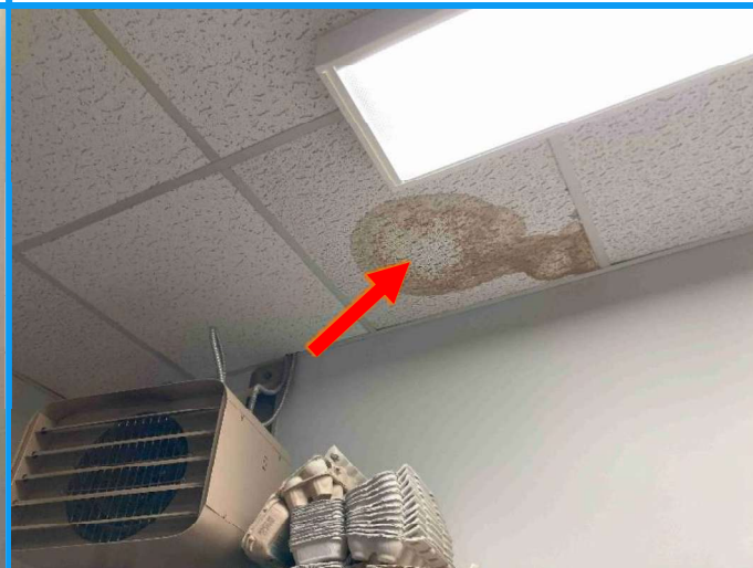
Photo 12: Typical view of the water-stained acoustic ceiling tile (see arrow) observed in the kitchen food prep area of the subject building.
