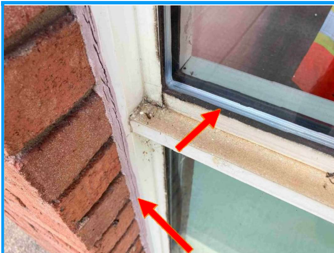
Photo 1: Typical view of the asbestos-containing black window glazing (see top arrow) and the non-asbestos containing light brown caulking (see bottom arrow) observed throughout the exterior of the subject building.
