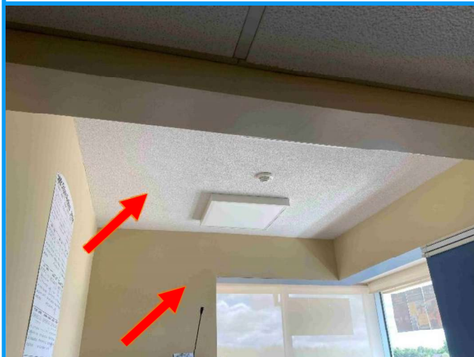
Photo 3: Typical view of the non-asbestos containing drywall walls (see bottom arrow) and the non-asbestos containing textured ceiling (see top arrow) in the subject building.
