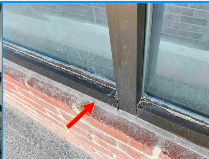
Photo 10: Typical view of the non-asbestos containing brown caulking on exterior window frame seams (see arrow).
