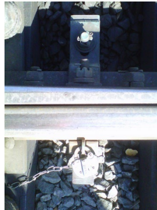
Figure SUB-PART D – 71 – Switch Point Foot Pedal Lock
