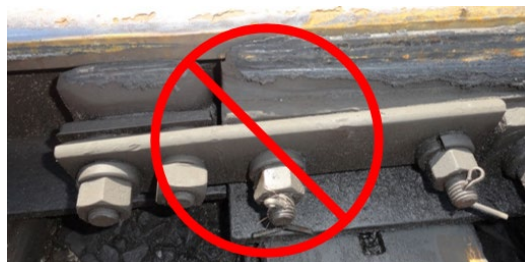
Figure SUB-PART D – 70 – Prohibited Switch Point Protector
