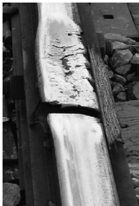
Figure SUB-PART D – 40 – Rail End Batter (left) and Straight Edge Placement (right)
