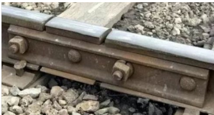
Figure SUB-PART D – 33 – Temporary Gap Rail Insert
