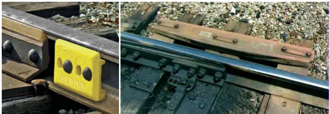
Figure SUB-PART D – 69 – Examples of Switch Point Protector and Guard
