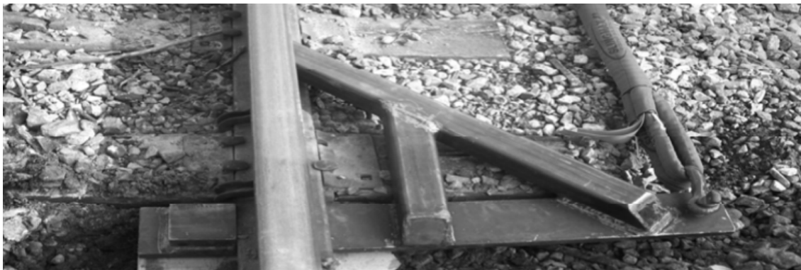
Figure SUB-PART D – 60 – Rail Grip (used to anchor rail to track structure)
