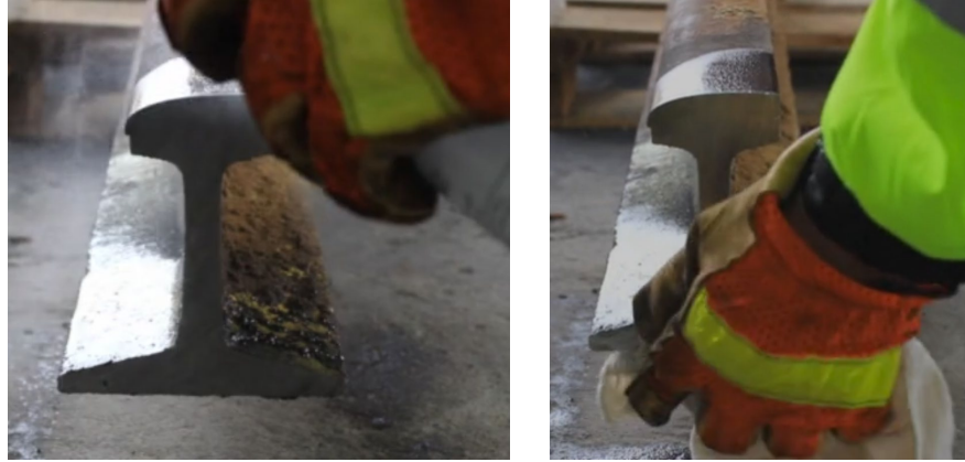
Figure SUB-PART D – 48 – Cleaning of Saw Cut Rail Surface
