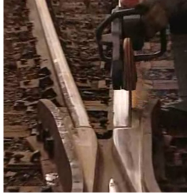
Figure Appendix M – 22 – SGM Frog – Slotting Mating Surfaces
