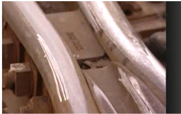
Figure Appendix M – 17 – RBM Frog – Flow Removed from Field Side at Frog Throat
