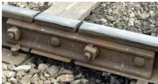
Figure SUB-PART D – 33 – Temporary Gap Rail Insert
