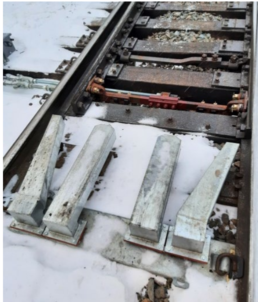
Figure Appendix N – 8 – Snow Clearing Operations / Cold Air Blower Nozzles
