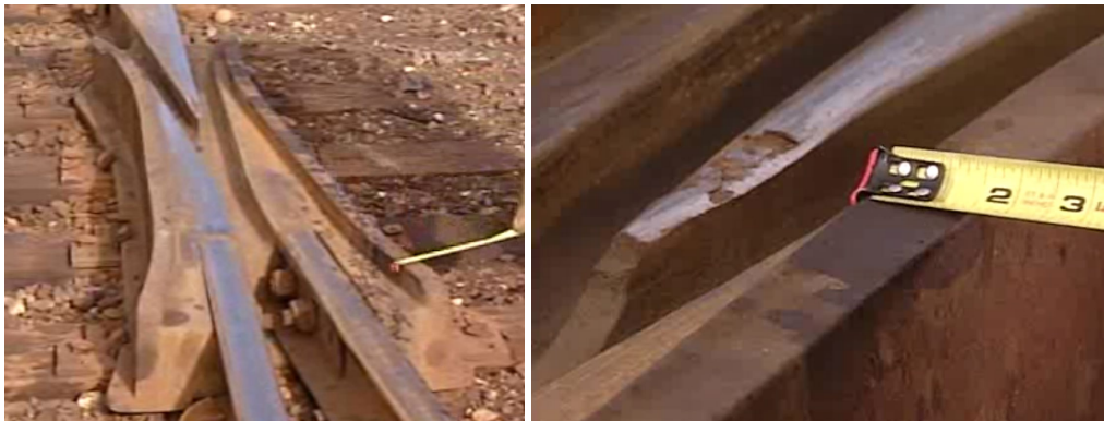
Figure Appendix M – 23 – SGM Frog – Guardrail Measurements
