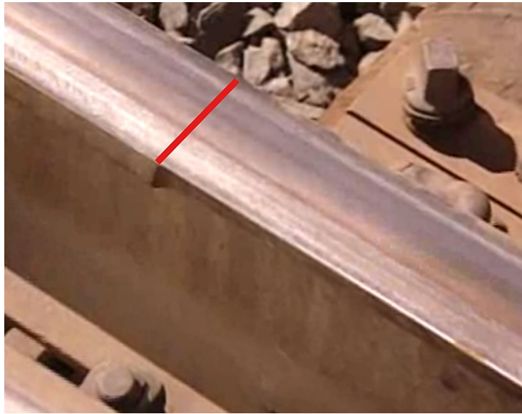
Figure Appendix M – 7 – Line Marking End of Undercut
