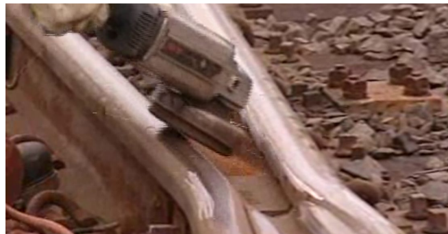
Figure Appendix M – 20 – RBM Frog – 9/16" (14 mm) Radius Restoration of Running Surfaces
