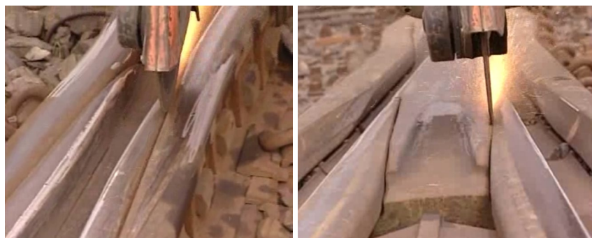
Figure Appendix M – 21 – RBM Frog – Slotting Mating Surfaces
