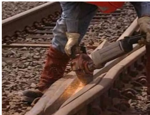
Figure Appendix M – 15 – RBM Frog – Grinding Frog Point and Wing Rails
