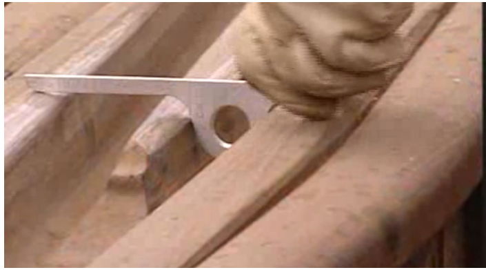
Figure Appendix M – 16 – RBM Frog – Flangeway Clearance Verification with Check Gauge
