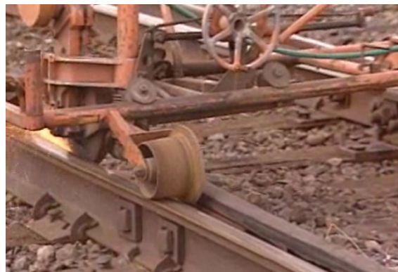
Figure Appendix M – 18 – RBM Frog – Flow Removed from Guard Rail Running Rail
