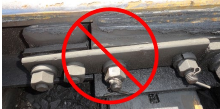
Figure SUB-PART D – 70 – Prohibited Switch Point Protector
