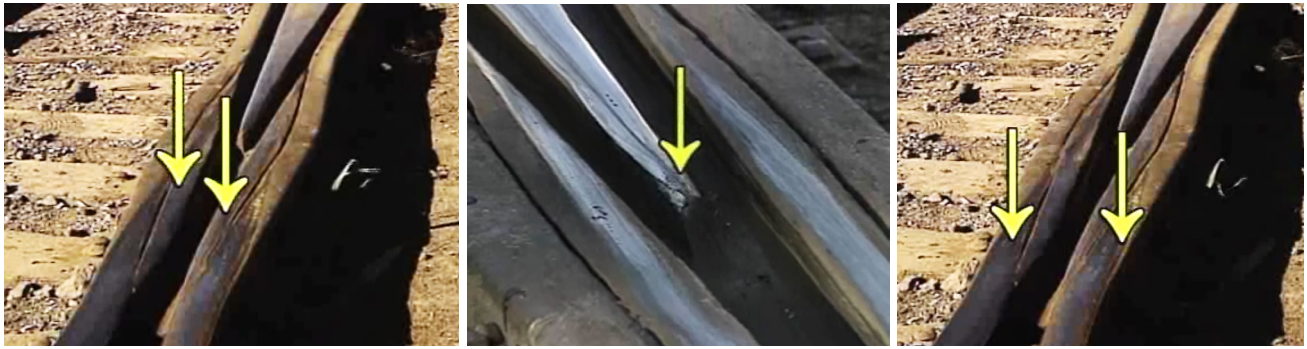
Figure Appendix M – 14 – RBM Frog – Wing Rails (left), Frog Point (centre) and Rails (right)
