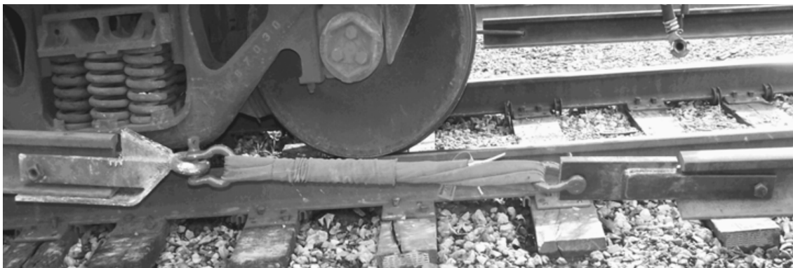
Figure SUB-PART D – 61 – End of One Rail Connected to the Beginning of Another Rail Being Unloaded
