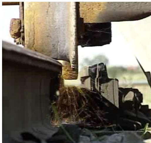
Figure Appendix M – 8 – Grinding of Standard Stock Rail
