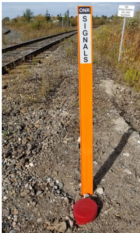
Figure Appendix N – 3 – Utility Marker
