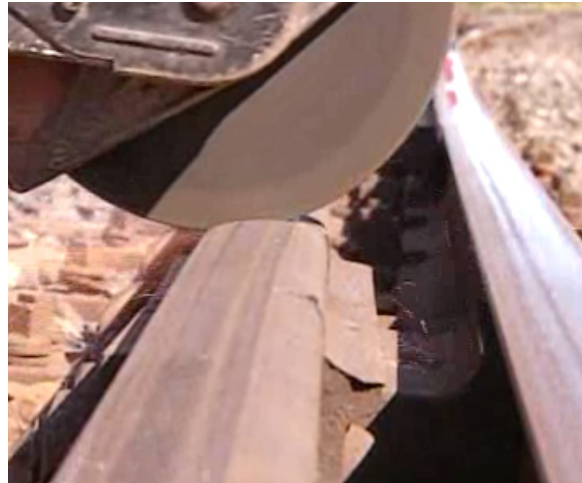
Figure Appendix M – 12 – Straight Slot at Heel Block
