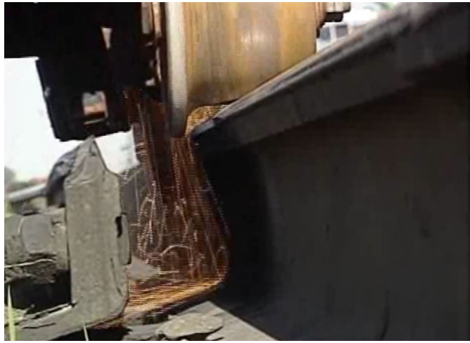
Figure Appendix M – 9 – Grinding of Undercut Stock Rail
