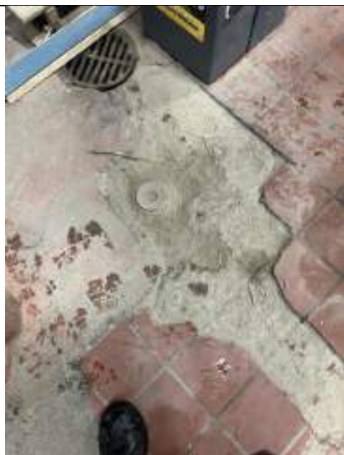
Picture 2.1 - Existing Flooring (Building North)
