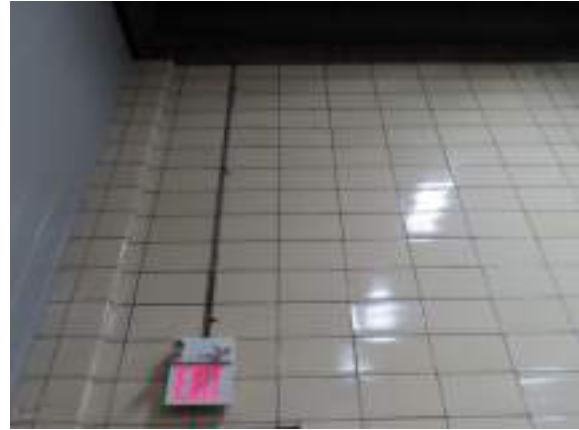
Cochrane Powerhouse - C301023
