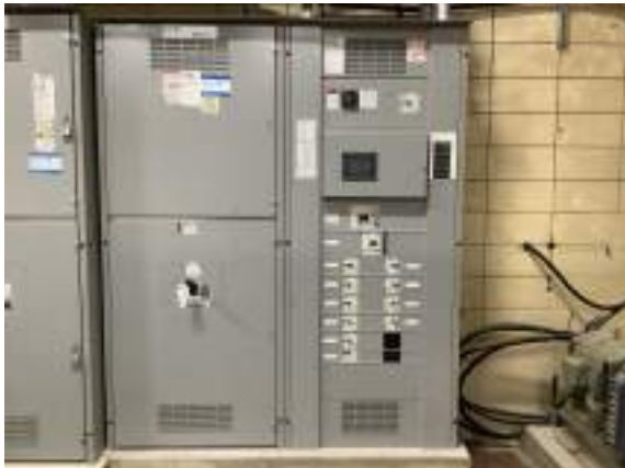
Cochrane Powerhouse - D501003
