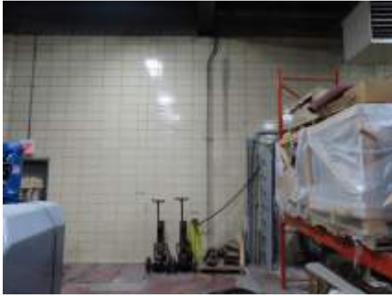
Cochrane Powerhouse - C301023
