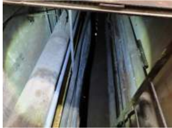
Cochrane Powerhouse - A101001
