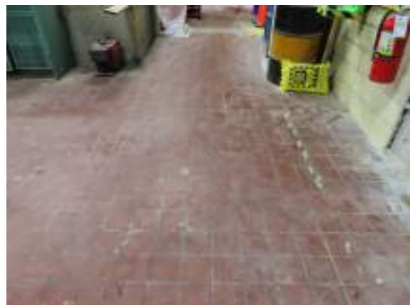
Cochrane Powerhouse - C302001
