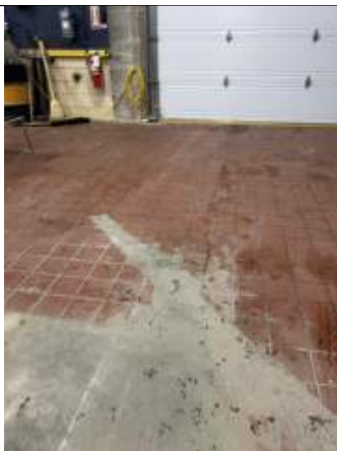
Picture 2.2 - Existing Flooring (BuildinNorth)
