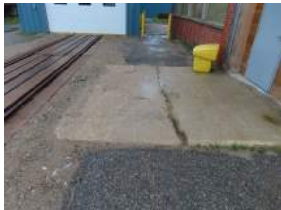
Cochrane Powerhouse - G202003
