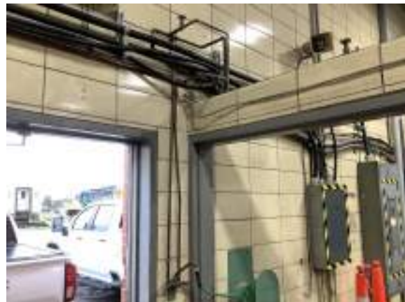
Cochrane Powerhouse - D202001
