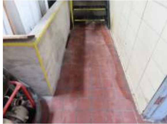
Cochrane Powerhouse - C302001
