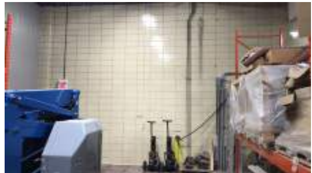
Cochrane Powerhouse - C301023
