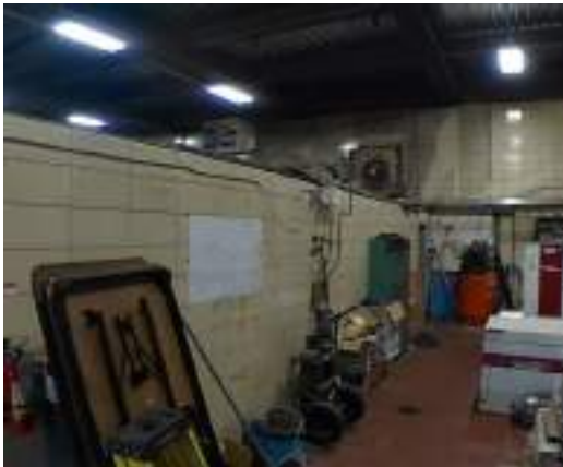
Cochrane Powerhouse - C101001
