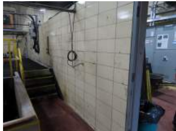
Cochrane Powerhouse - C301023
