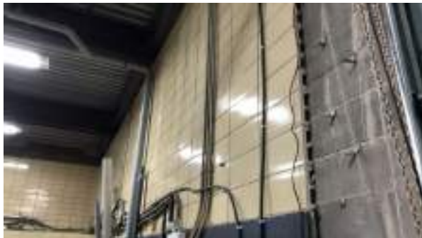
Cochrane Powerhouse - C301023
