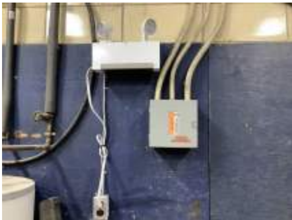
Cochrane Powerhouse - D509003
