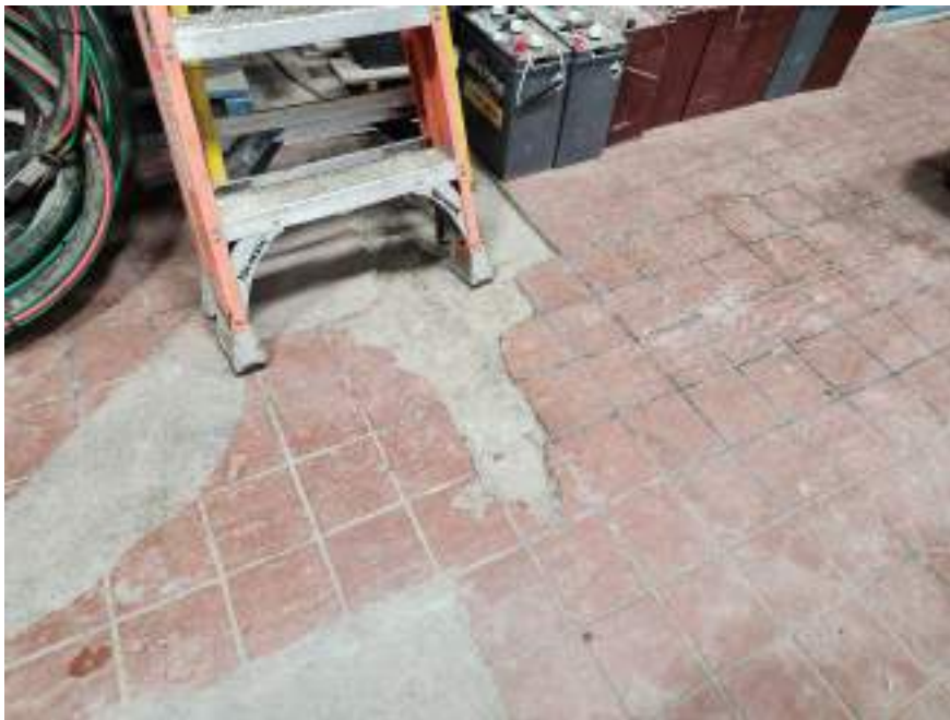
Figure 8: Flooring defects
