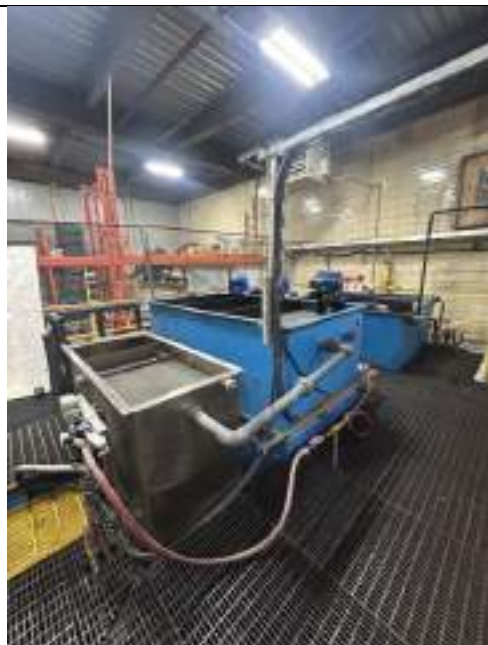
Picture 1.3 - Overall Photo (Building Central)
