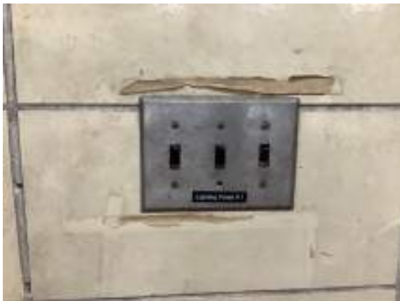
Cochrane Powerhouse - D502001
