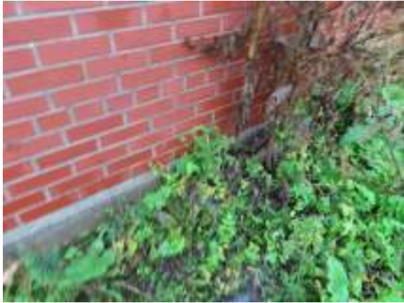
Cochrane Powerhouse - A101001
