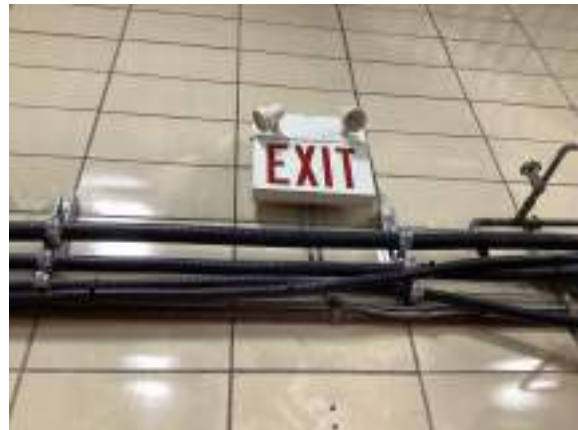
Cochrane Powerhouse - D502003
