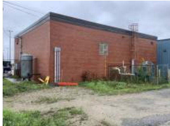
Cochrane Powerhouse - D301002
