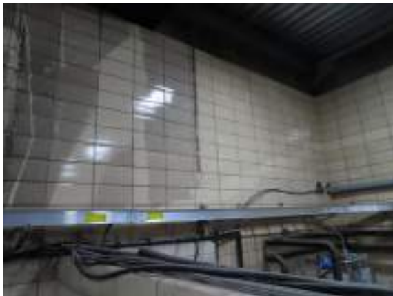
Cochrane Powerhouse - C301023
