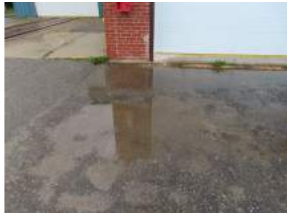
Cochrane Powerhouse - G202003
