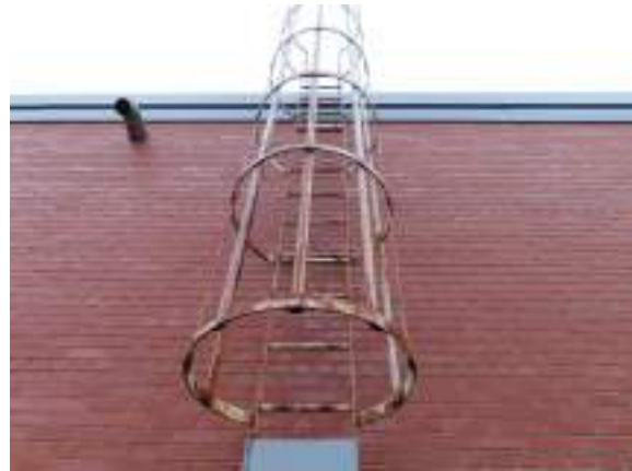
Cochrane Powerhouse - C201002
