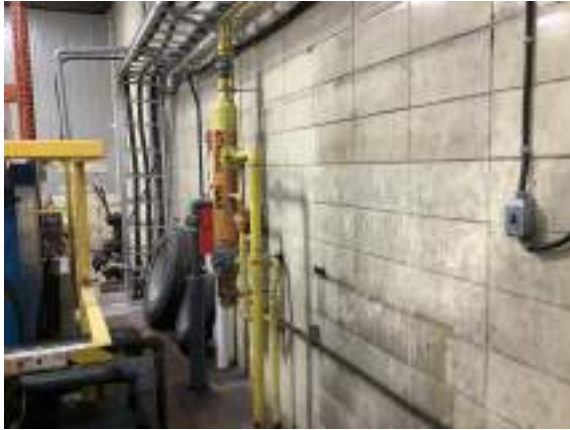
Cochrane Powerhouse - D301002
