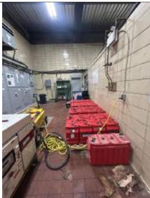
Picture 1.9 - Overall Photo (Building South)
