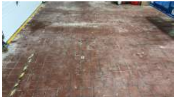
Cochrane Powerhouse - C302001
