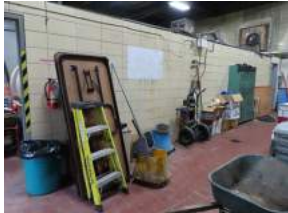
Cochrane Powerhouse - C101001
