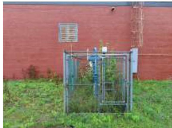
Cochrane Powerhouse - G204001
