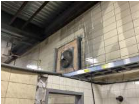
Cochrane Powerhouse - D304007
