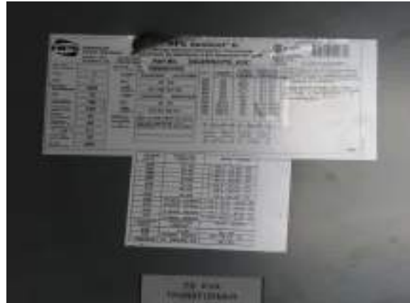
Cochrane Powerhouse - D501002
