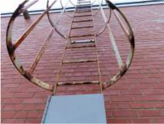
Cochrane Powerhouse - C201002
