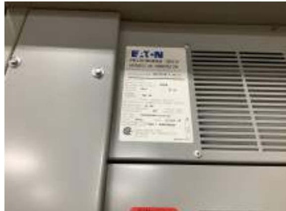
Cochrane Powerhouse - D501003
