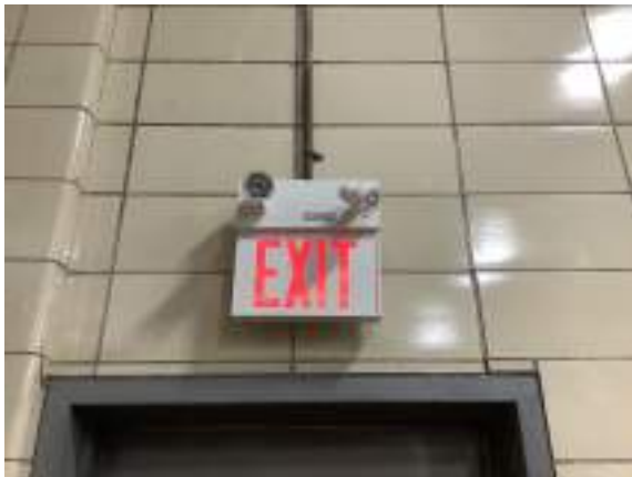
Cochrane Powerhouse - D502003
