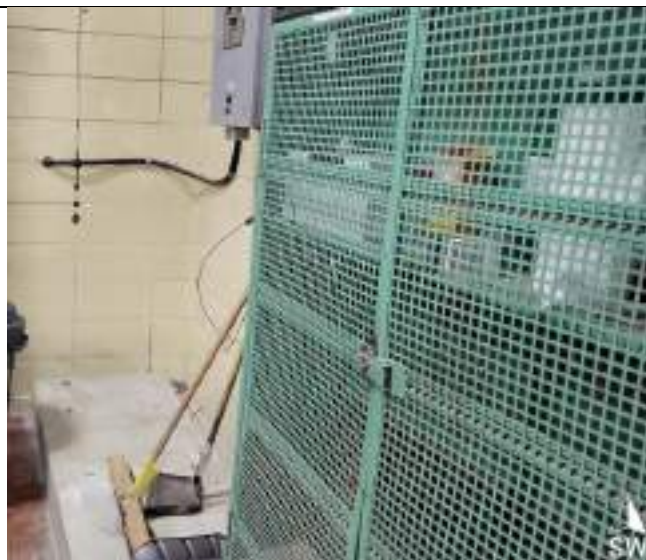
Picture 4.7 - Concrete Pad
