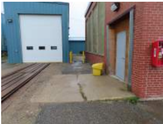
Cochrane Powerhouse - G202003
