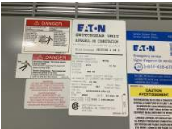
Cochrane Powerhouse - D501003
