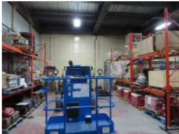
Cochrane Powerhouse - C301023
