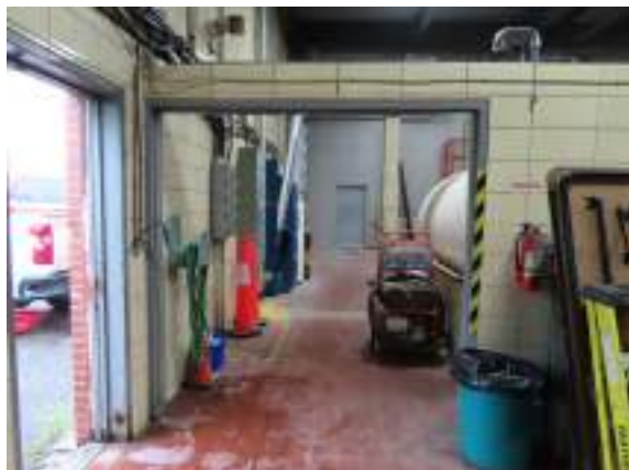
Cochrane Powerhouse - C101001
