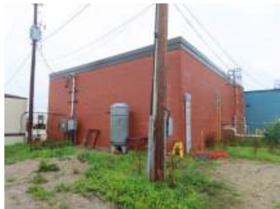
Cochrane Powerhouse - G205004
