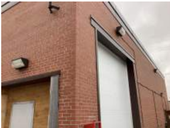
Cochrane Powerhouse - D502041
