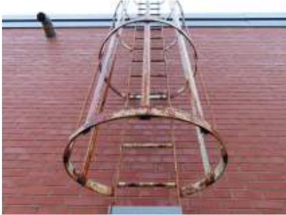
Cochrane Powerhouse - C201002
