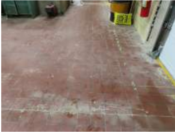
Cochrane Powerhouse - C302001
