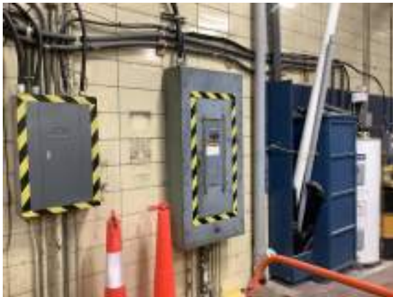
Cochrane Powerhouse - D501005
