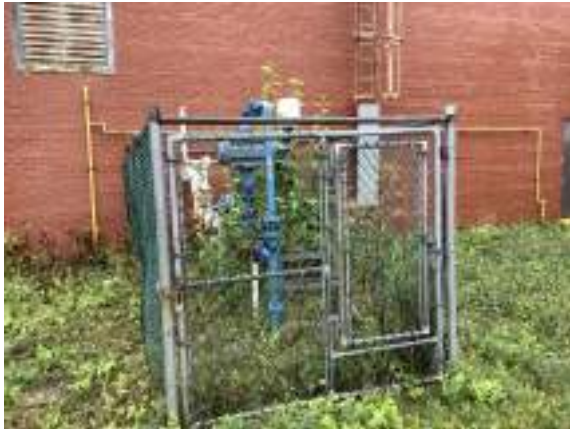
Cochrane Powerhouse - D301002
