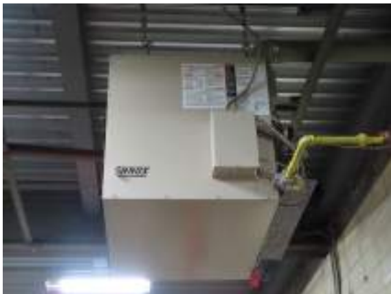
Cochrane Powerhouse - D305002
