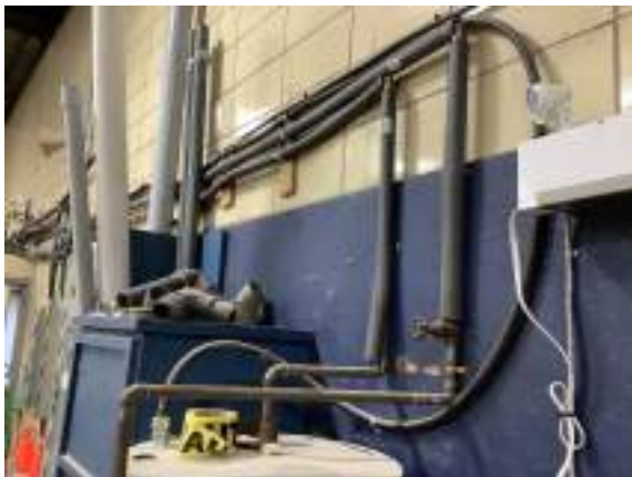
Cochrane Powerhouse - D202001
