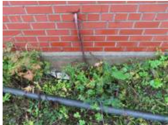
Cochrane Powerhouse - A101001
