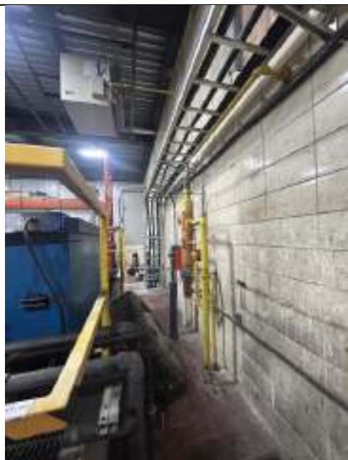
Picture 1.5 - Overall Photo (Building Central)
