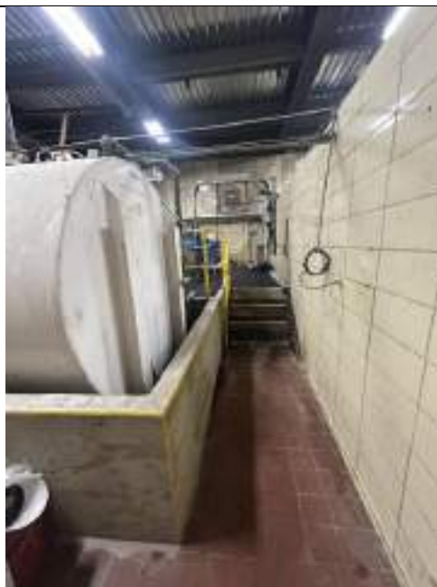
Picture 1.6 - Overall Photo (Building Central)
