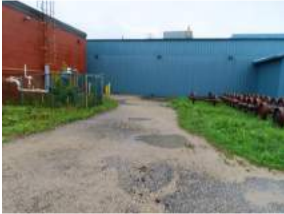
Cochrane Powerhouse - G202003
