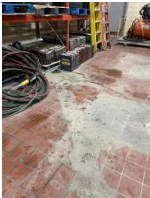
Picture 2.3 - Existing Flooring (Building North)
