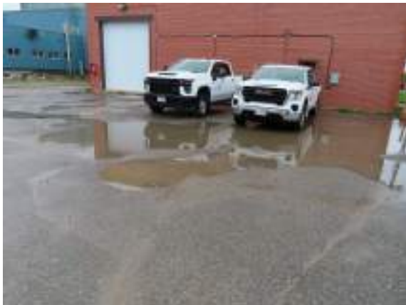
Cochrane Powerhouse - G202003
