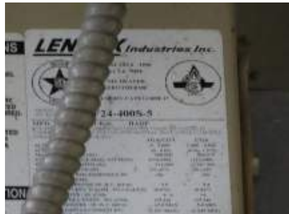
Cochrane Powerhouse - D305002
