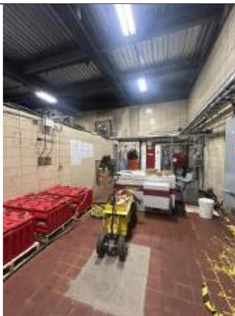
Picture 1.8 - Overall Photo (Building South)
