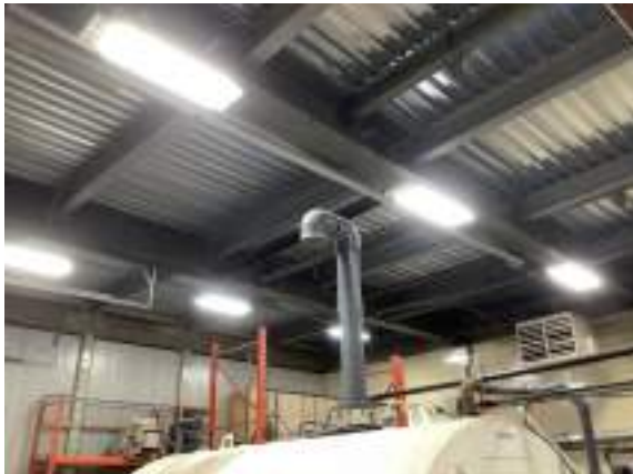
Cochrane Powerhouse - D502002
