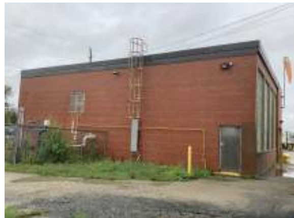
Cochrane Powerhouse - D502041
