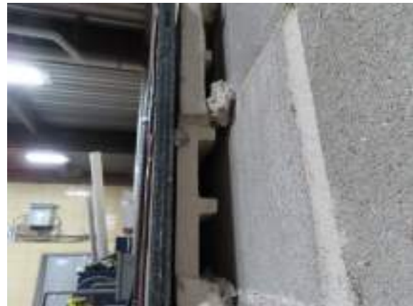
Cochrane Powerhouse - C301023
