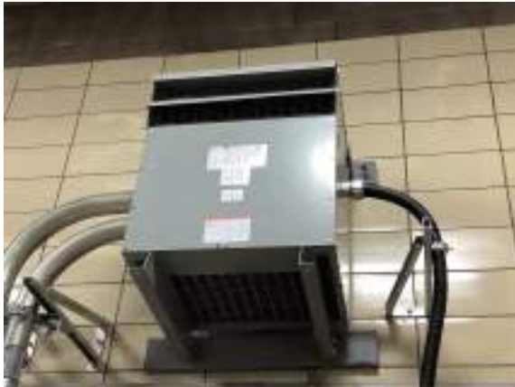
Cochrane Powerhouse - D501002
