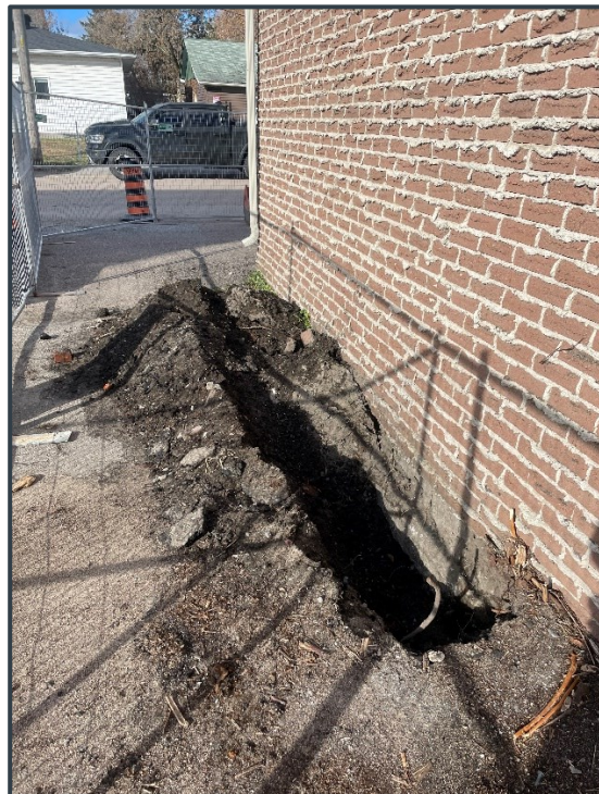
Photograph 2: Displaying the stockpile on the northwest side of the building
