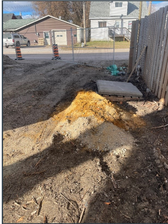
Photograph 3: Displaying the stockpile on the southeast side of the building
