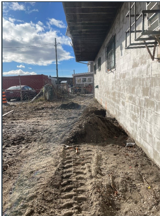
Photograph 4: Displaying the stockpile on the southwest side of the building
